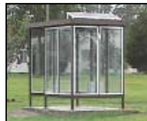
Solar powered shelter
