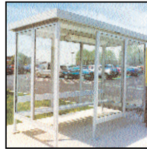
Mass transit bus shelter
